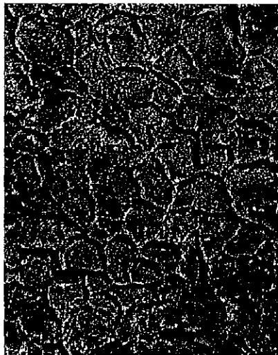
PLATE 12 TOP SURFACE SHOWING HEAVILY CRACKED GRAY COATING MATERIAL AND A FEW EXPOSED FINE AGGREGATE PARTICLES
