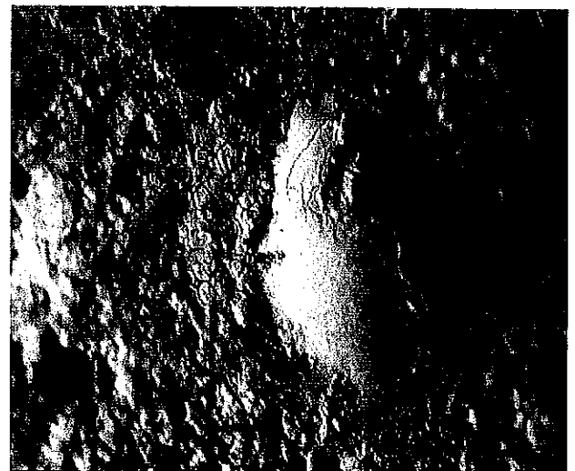
PLATE 6 CORE EDGE SURFACE SHOWING PARTIALLY CRACKED ALKALIC GEL EXUDATIONS
