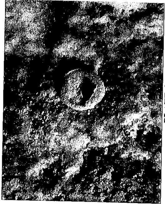
PLATE 6 CUT SURFACE "103TUD-P" SHOWING CRACKED GEL "BUBBLE" EXUDATION
