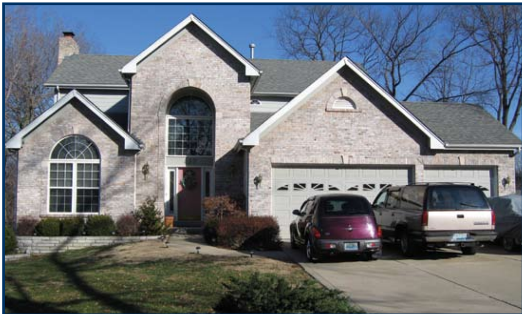
A "blighted" home in Sunset Hills.
